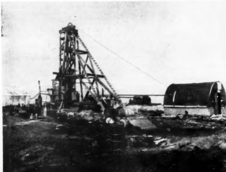
LEFT: The pre-fabricated headframe is bolted together to facilitate transportation and erection. RIGHT: Two miners lowered to the 125-foot level new sinter machine and a second will be added in the relatively near future.
